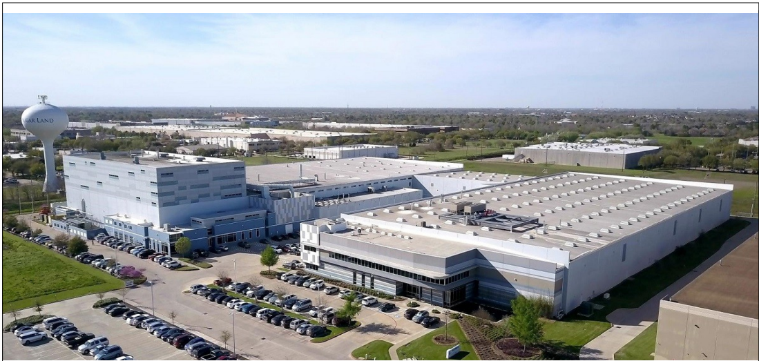
Accredo's 550,000-sq-ft greenfield plant in Sugar Land, Texas, is designed and built to LEED certification standards and houses some of the most sophisticated converting equipment available.
