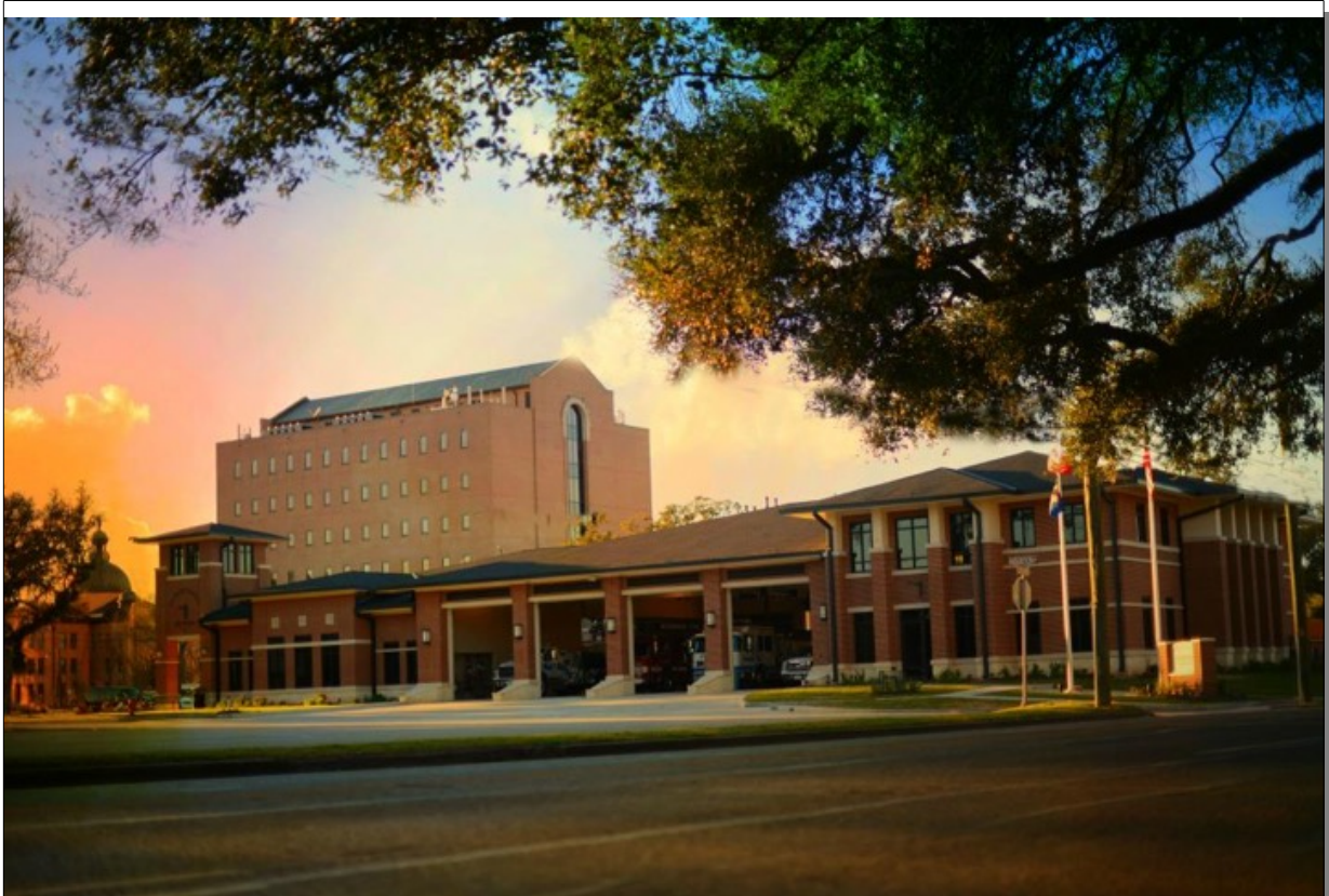
City of Richmond Fire Station #1, 200 Houston St., Richmond, Texas
