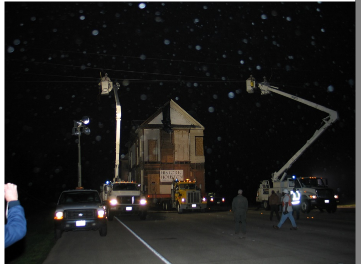
CenterPoint Energy directed the highway move, with TXDOT concurrence, to assure public safety as well as the safety of the contractor and for the protection of the house.
