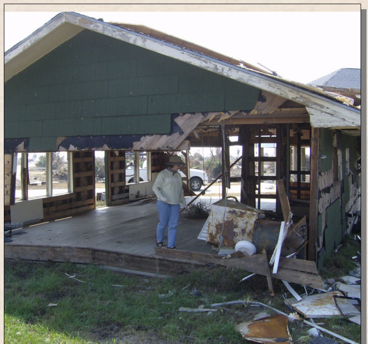
Repairing Jane's house on Bolivar Peninsula
