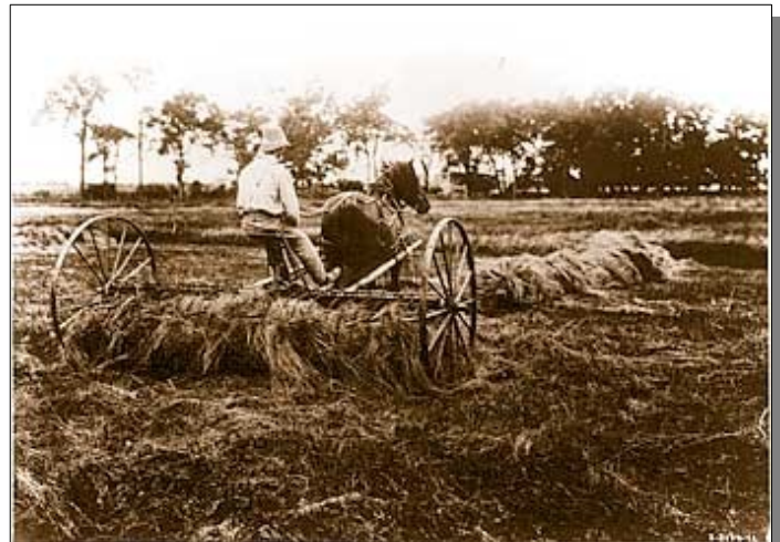
A dump rake is a hay rake mounted on two wheels consisting of a set of long curved steel teeth and equipped with a device for raising the teeth to dump the hay. A horse or mule did most of the work.
